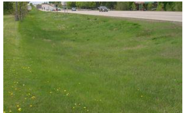
Photo of a well-maintained dry swale. Courtesy of Limnotech.
