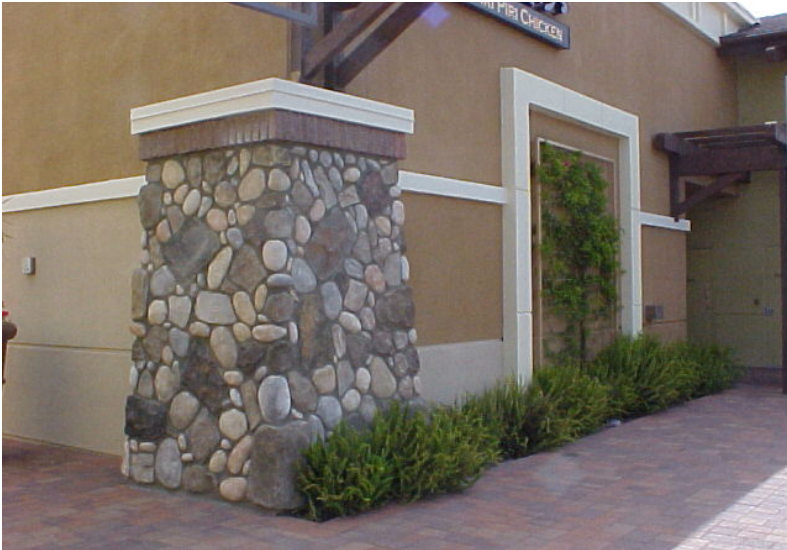
An encouraged “back of building” architectural detail
