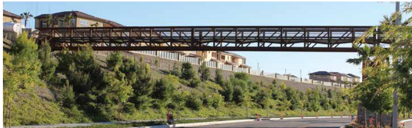
New Alton Parkway Pedestrian Bridge
